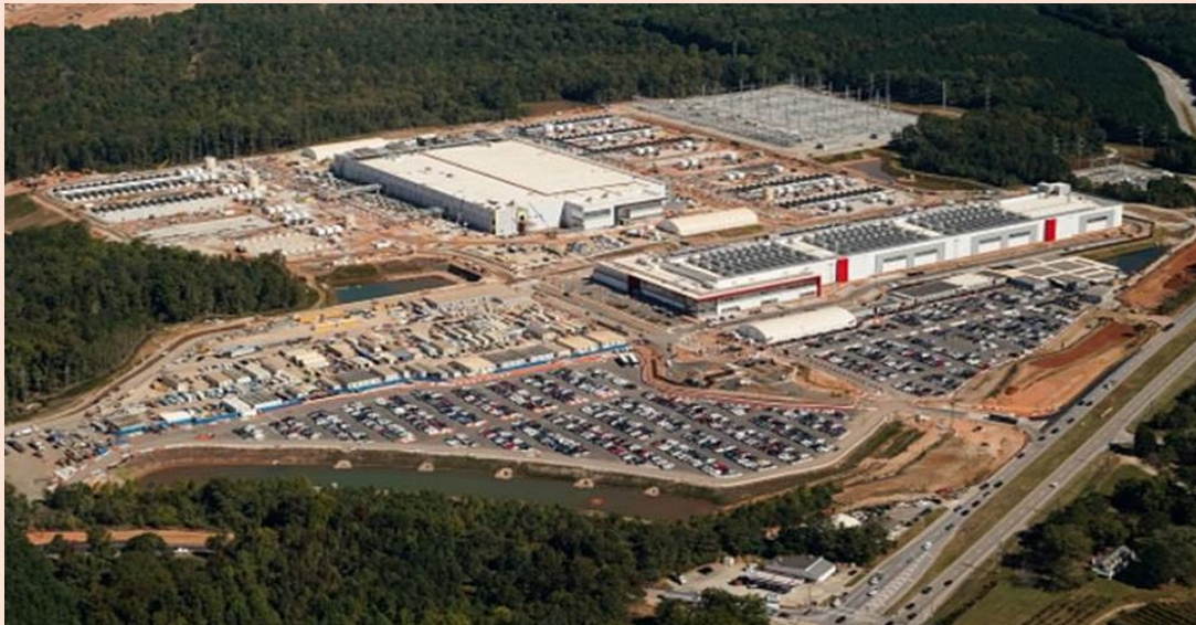
The enormous QTS data center development project in Fayetteville, Georgia.
