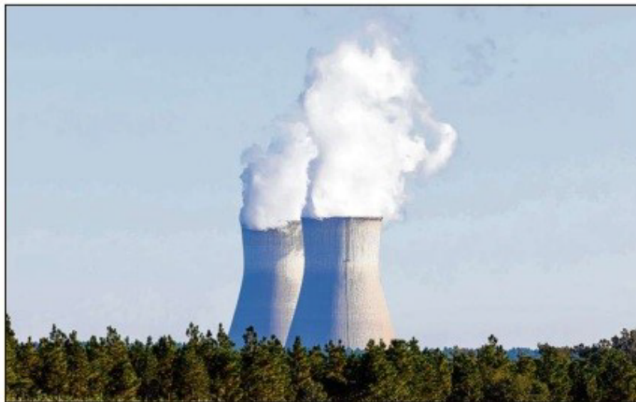
Cooling tower units 1 and 2 of Plant Vogtle in Burke County are seen in October. Vogtle's units 3 and 4 remain the only nuclear-plant construction in the entire nation and have already cost nearly two-and-a-half times the price promised, and a six-year project is now seven years behind schedule. ARVIN TEMKAR/AJC 2022
